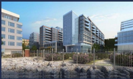
Building 9 at Port Imperial- Weehawken, NJ (In-Construction)
