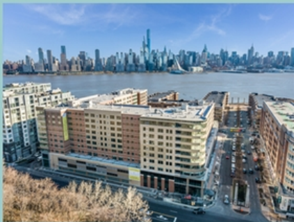
The Capstone – West New York, NJ (In-Construction)
