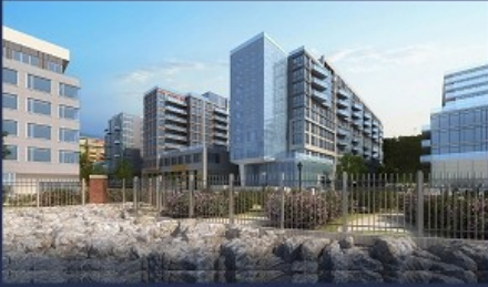
RiverHouse 9 - Weehawken, NJ (In-Construction)
