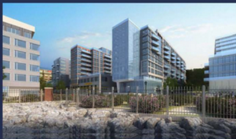
Building 9 at Port Imperial- Weehawken, NJ (In-Construction)
