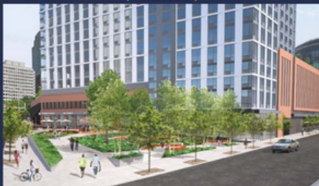
The Charlotte - Jersey City, NJ (In-Construction)
