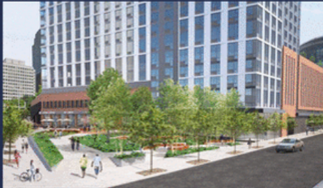
The Charlotte - Jersey City, NJ (In-Construction)
