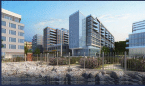
Building 9 at Port Imperial- Weehawken, NJ (In-Construction)
