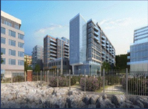
Building 9 at Port Imperial- Weehawken, NJ (In-Construction)
