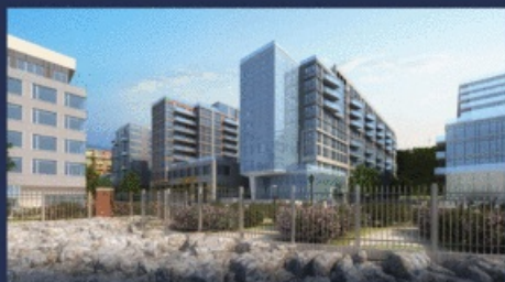
Building 9 at Port Imperial- Weehawken, NJ (In-Construction)
