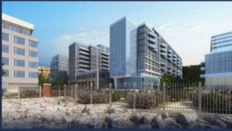
Building 9 at Port Imperial- Weehawken, NJ (In-Construction)
