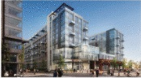
RiverHouse 11 at Port Imperial (295 Units) 2Q 2018 Delivery
