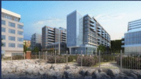
Building 8/9 at Port Imperial- Weehawken, NJ (In-Construction)
