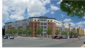
145 Front Street at City Square (365 Units) 1Q 2018 Delivery
