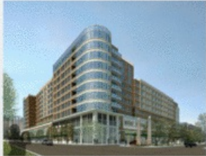
PI North – Riverwalk C
