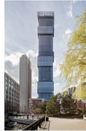
Urby at Harborside - 762 units 36% leased (275 units)
