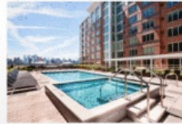
RiverTrace at Port Imperial West New York, NJ Stabilized
