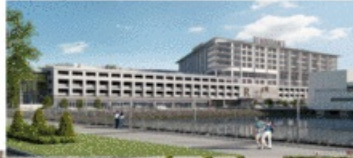
PI Hotel – 372 Keys In-Construction
