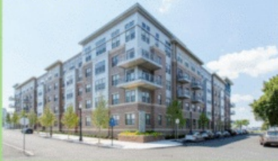
Portside at East Pier
