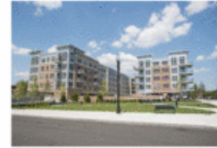
Portside at East Pier
