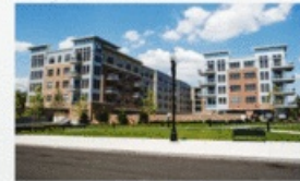
Portside at East Pier
