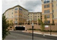
Highlands at Morristown Station 217 Units (Operating) 25% Ownership Prudential, Woodmont
